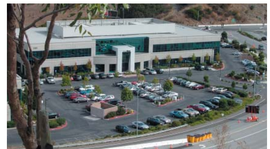
Parking lot, Sierra Point.
