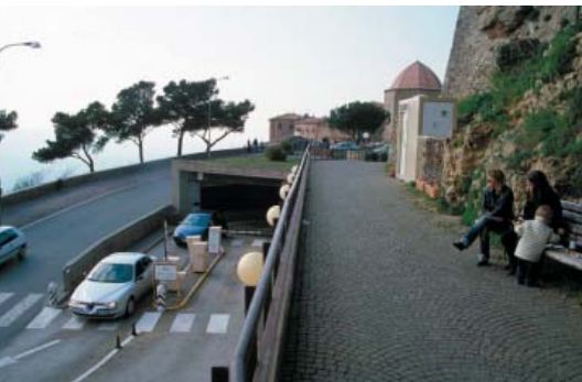
A buried parking garage under a park.
