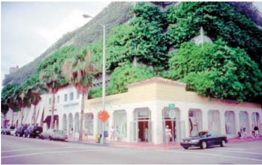
Covered parking structure.
