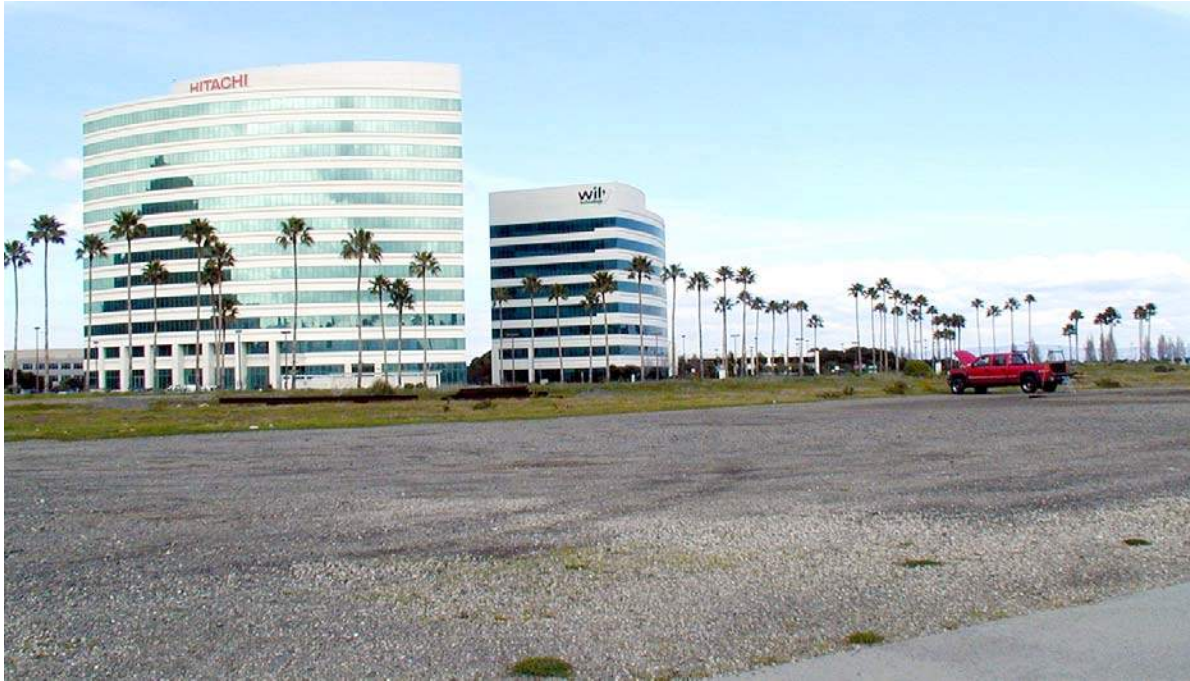
Photo 1: View looking northeast of Bay Trail and gravel parking area on the project site (foreground) and adjacent office buildings (background).
