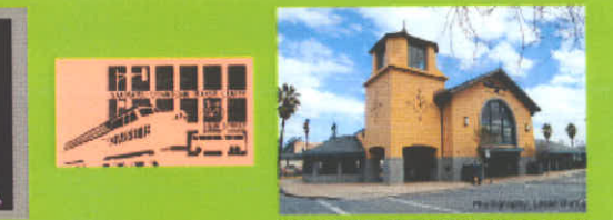
SAN MATEO TRANSIT CENTER 2009 DEDICATION 2009
