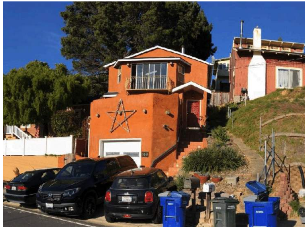
EXISTING FRONT FACADE - VIEW FROM SANTA CLARA STREET
