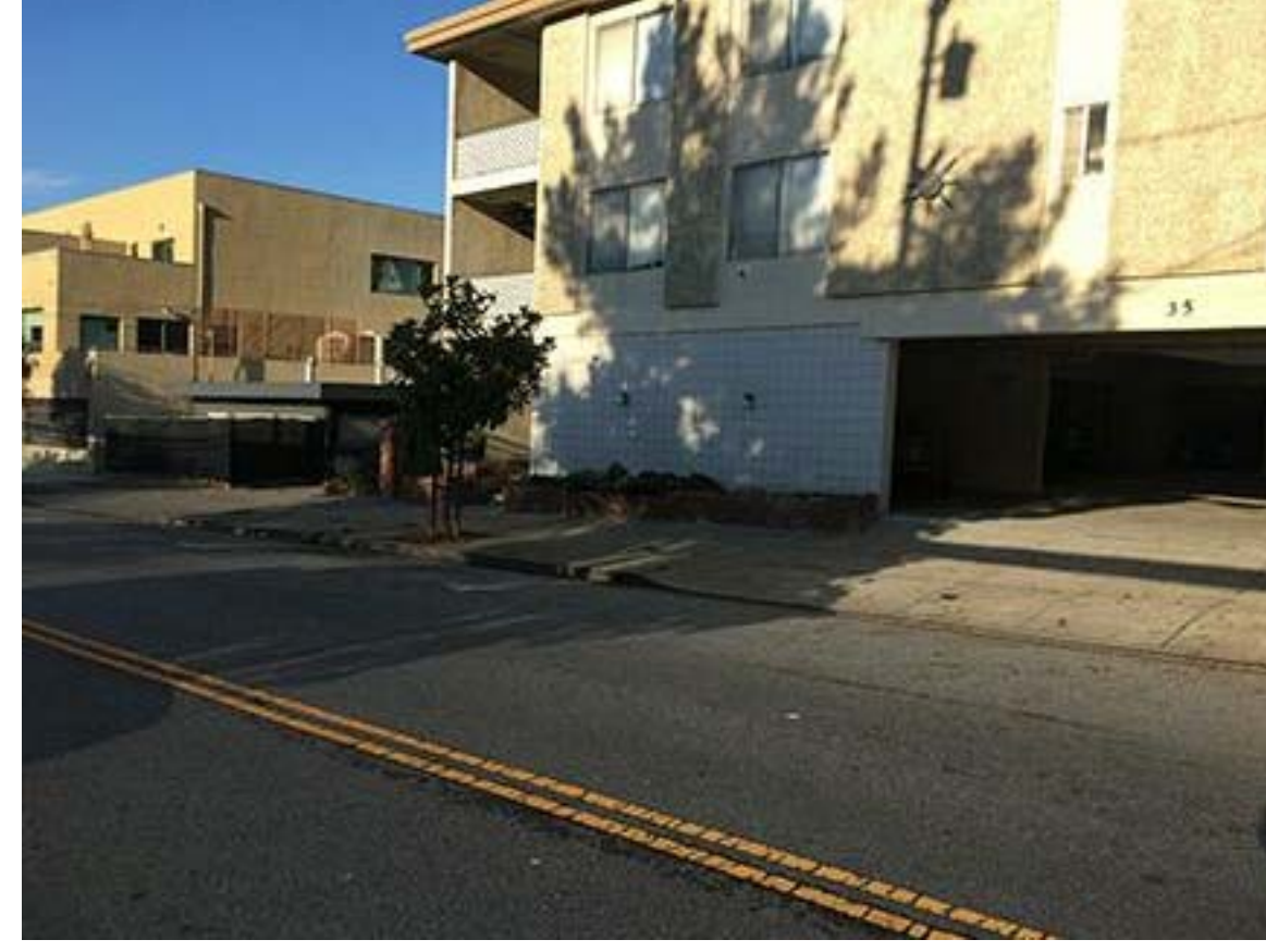
17 - VIEW ACROSS THE STREET
