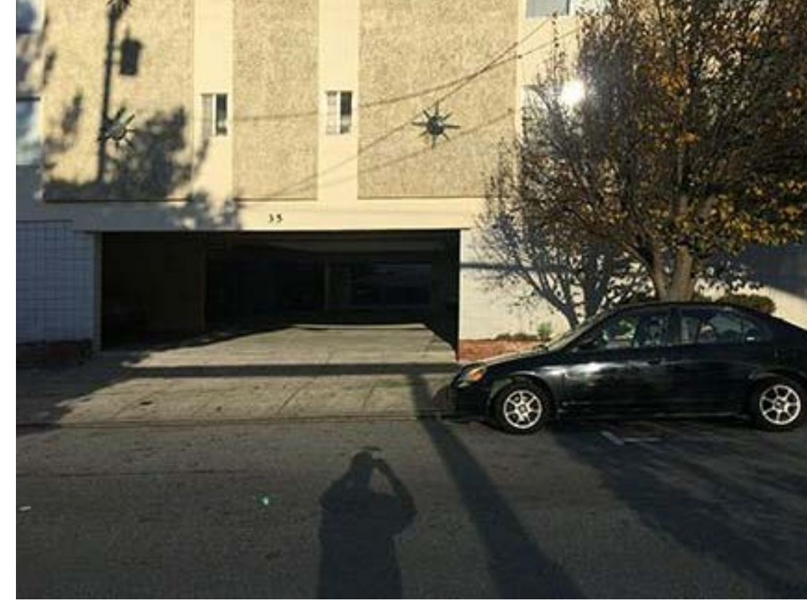
18 - VIEW ACROSS THE STREET
