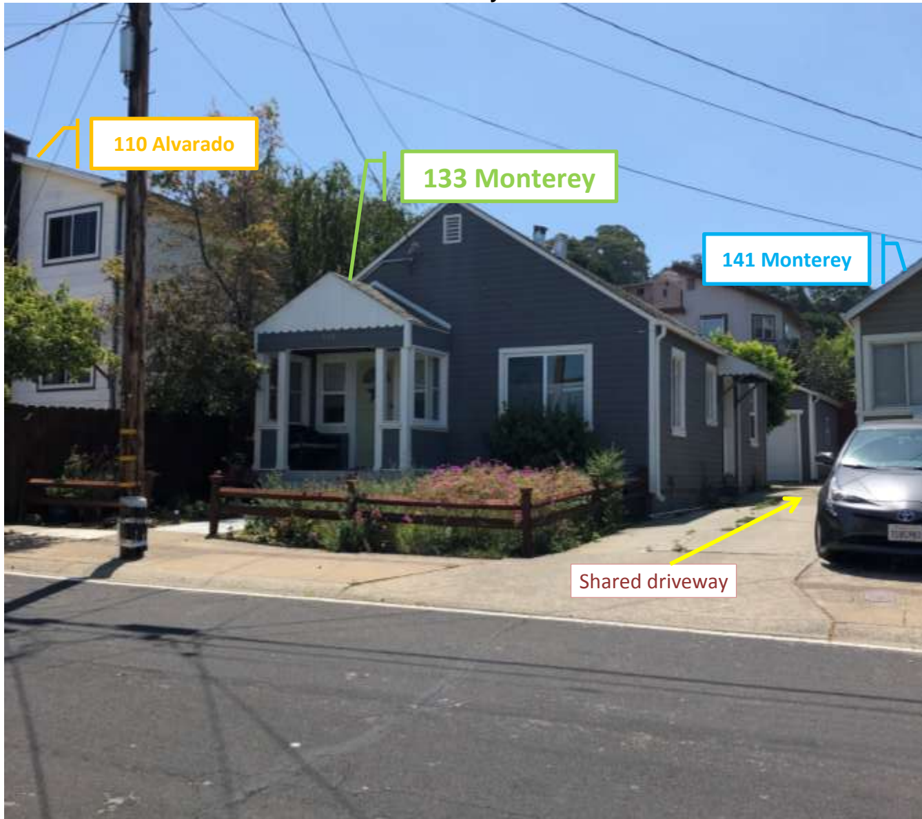
View from Monterey St (100-block, even) looking south at subject property
