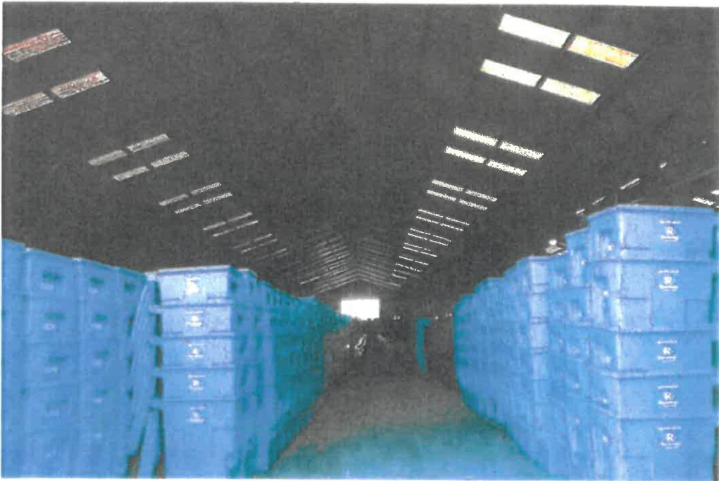
Building 3, interior, looking east
