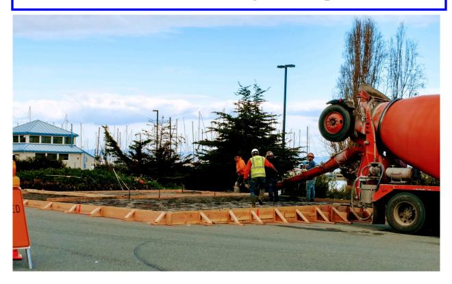
Here we are pouring the foundation for the NEW marina workshop building, which we had to locate in a much higher elevation on the property due to the newest sea level map projections from FEMA. This structure will enable us to safely and efficiently repair the many items we build or fix annually.
