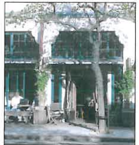
Storefront with punched openings and transoms
