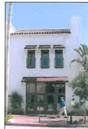
Storefront accented with awnings and simple chimney
