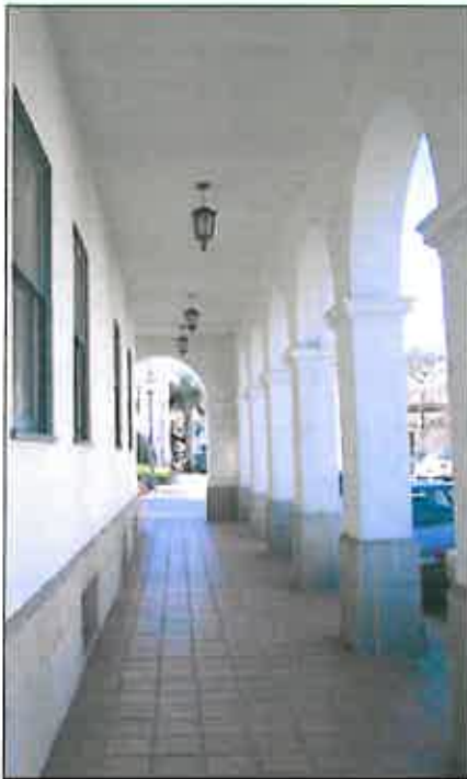
Loggia with arcade along street
