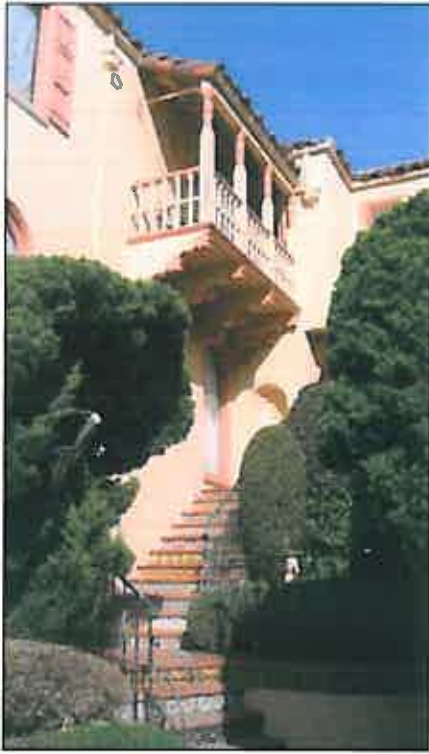
Exterior stair leading to entry door
