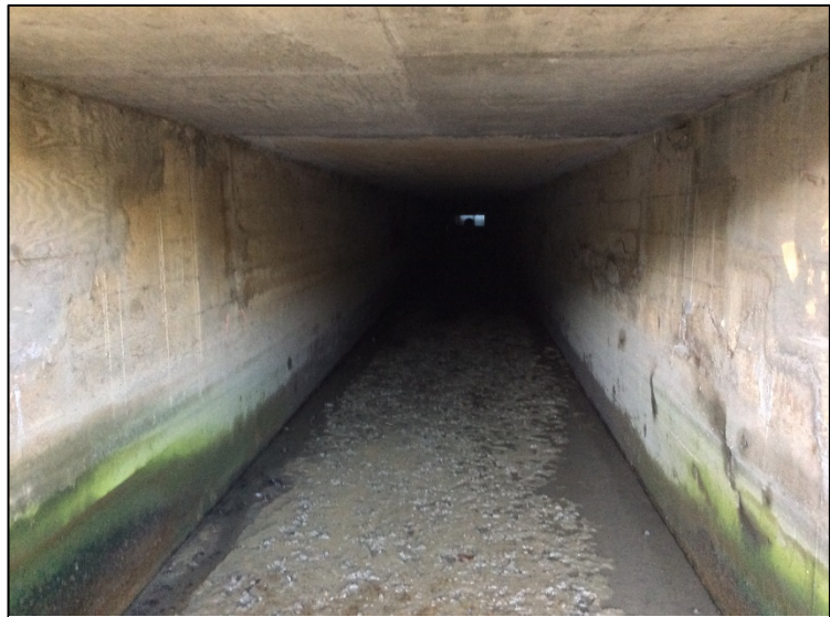
Photo 4. Concrete box culvert
