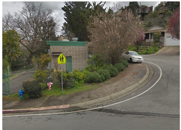
8. Pump Station at Lake Street & Glen Park Way
