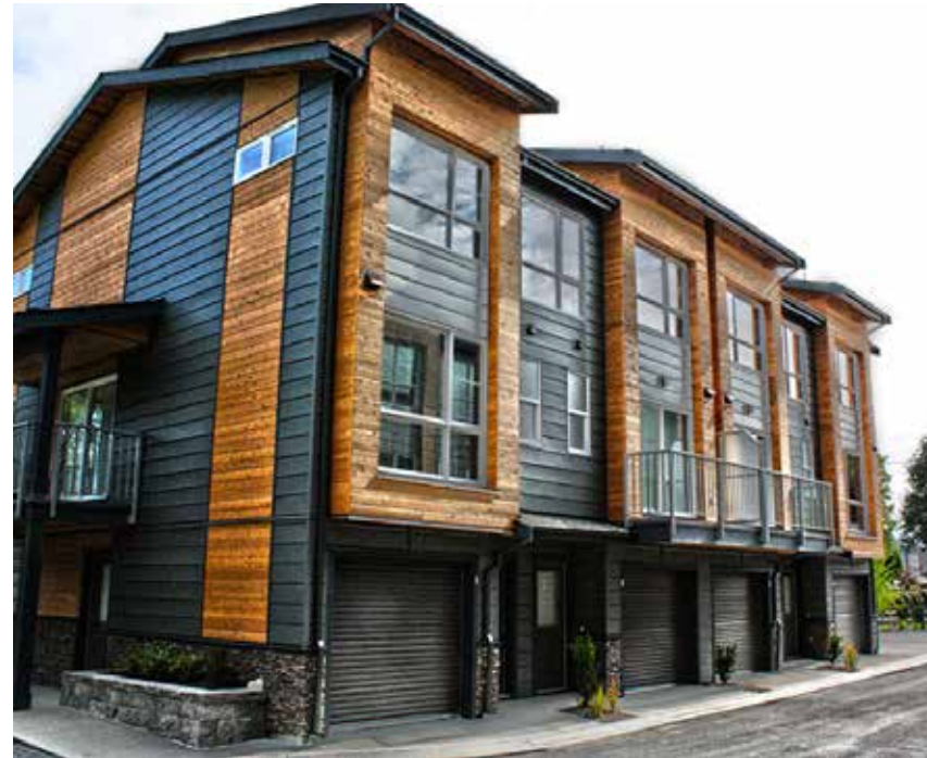
Garage doors shall have an equivalent or greater setback as the predominant building wall.
