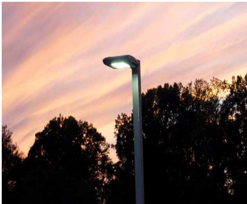
Lighting should be Dark Sky compliant and designed to accommodate both vehicles and pedestrians.
