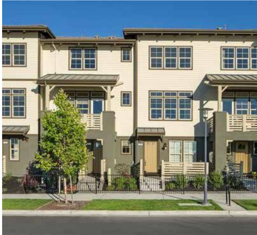
Residential building design should incorporate outdoor space, entryway transitions, and architectural variation.
