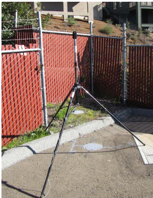
Site 989 –Golden Aster Pump Station
