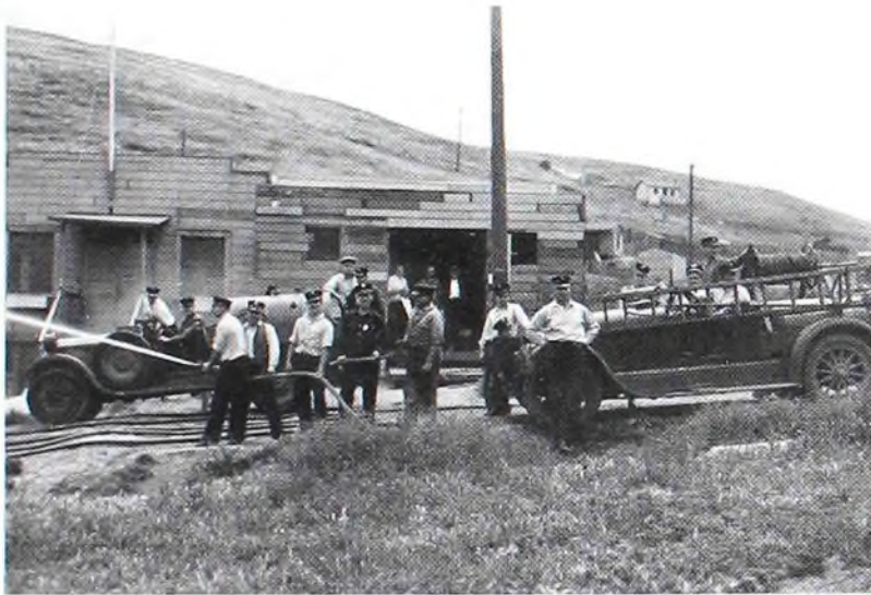
Two drills were on the agenda this date in 1933. Here the volunteers have run hose and spray in front of the social hall at Alvarado and San Bruno avenues. An addition to the social hall is under construction in the background. Mascot Louise Terry is at center.
