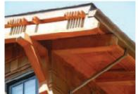
Building with copper flashing, gutter and drainpipe.
