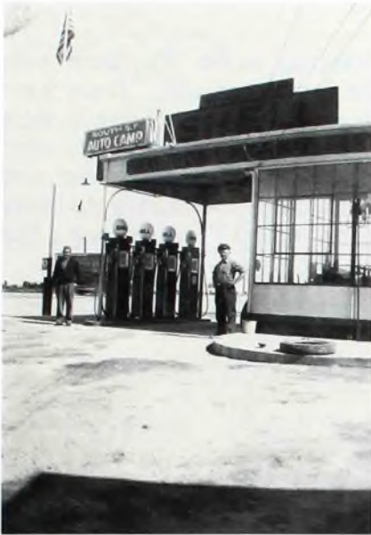
The Mozzetti's gas station --1939
