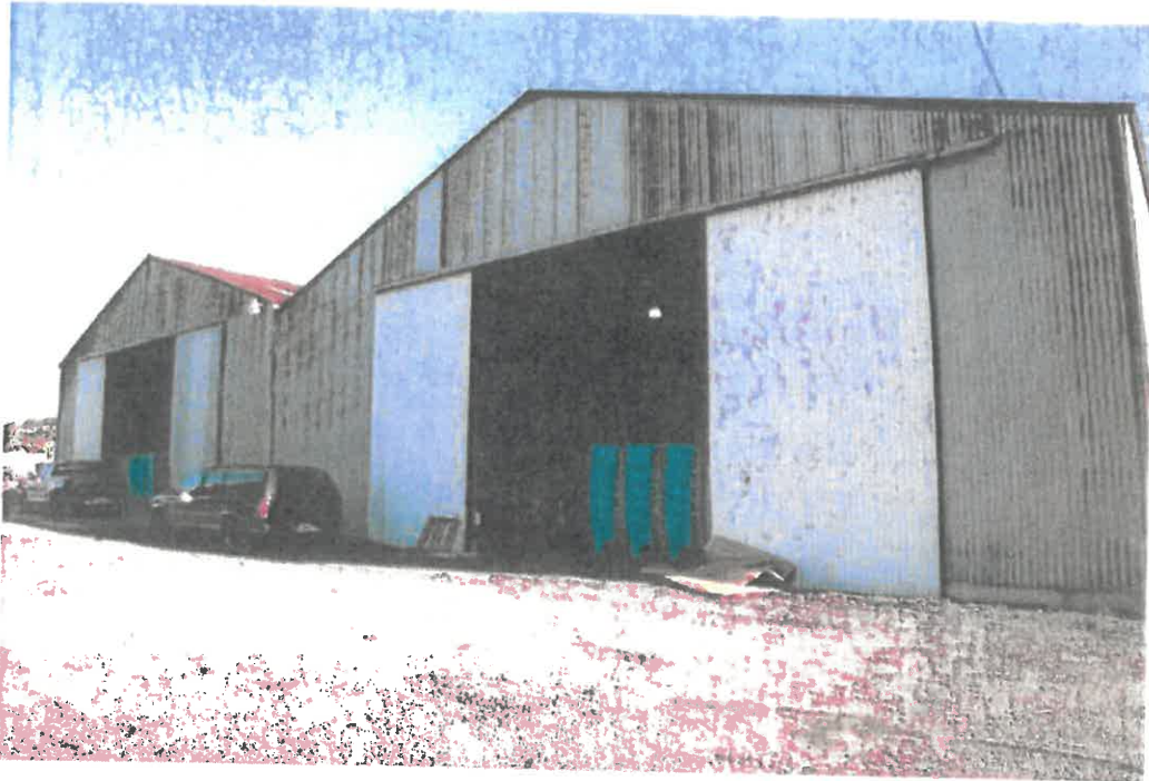
Buildings 3 and 4, west façade
