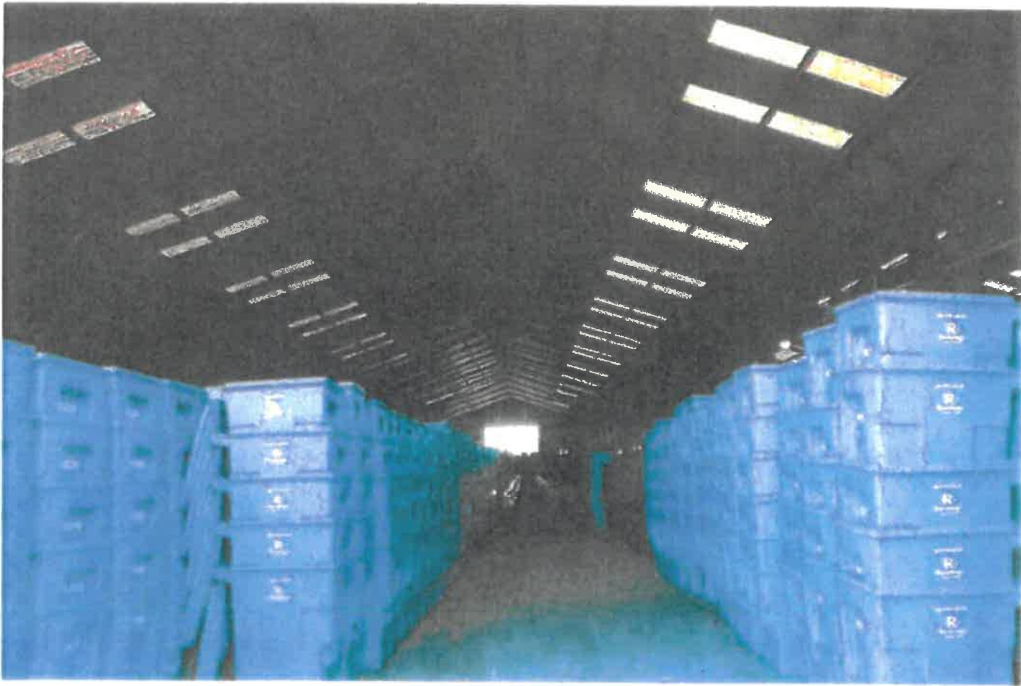
Building 3, interior, looking east
