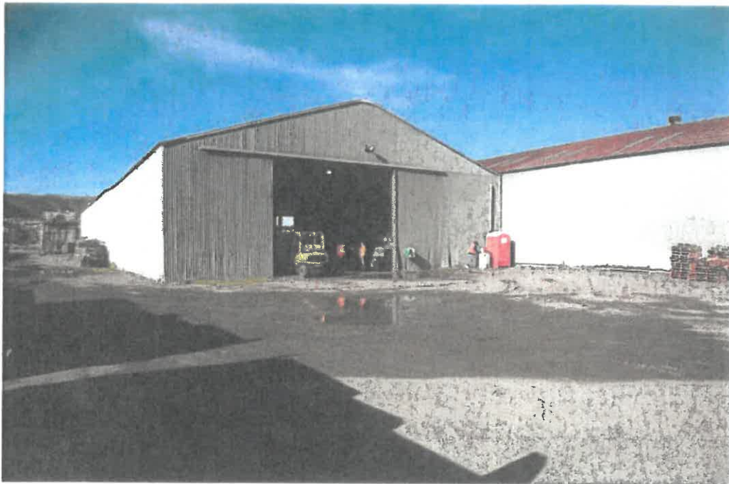
Building 4, east and south facades
