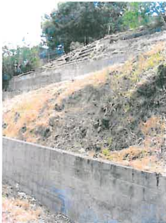
EXISTING RETAINING WALL PHOTOS
