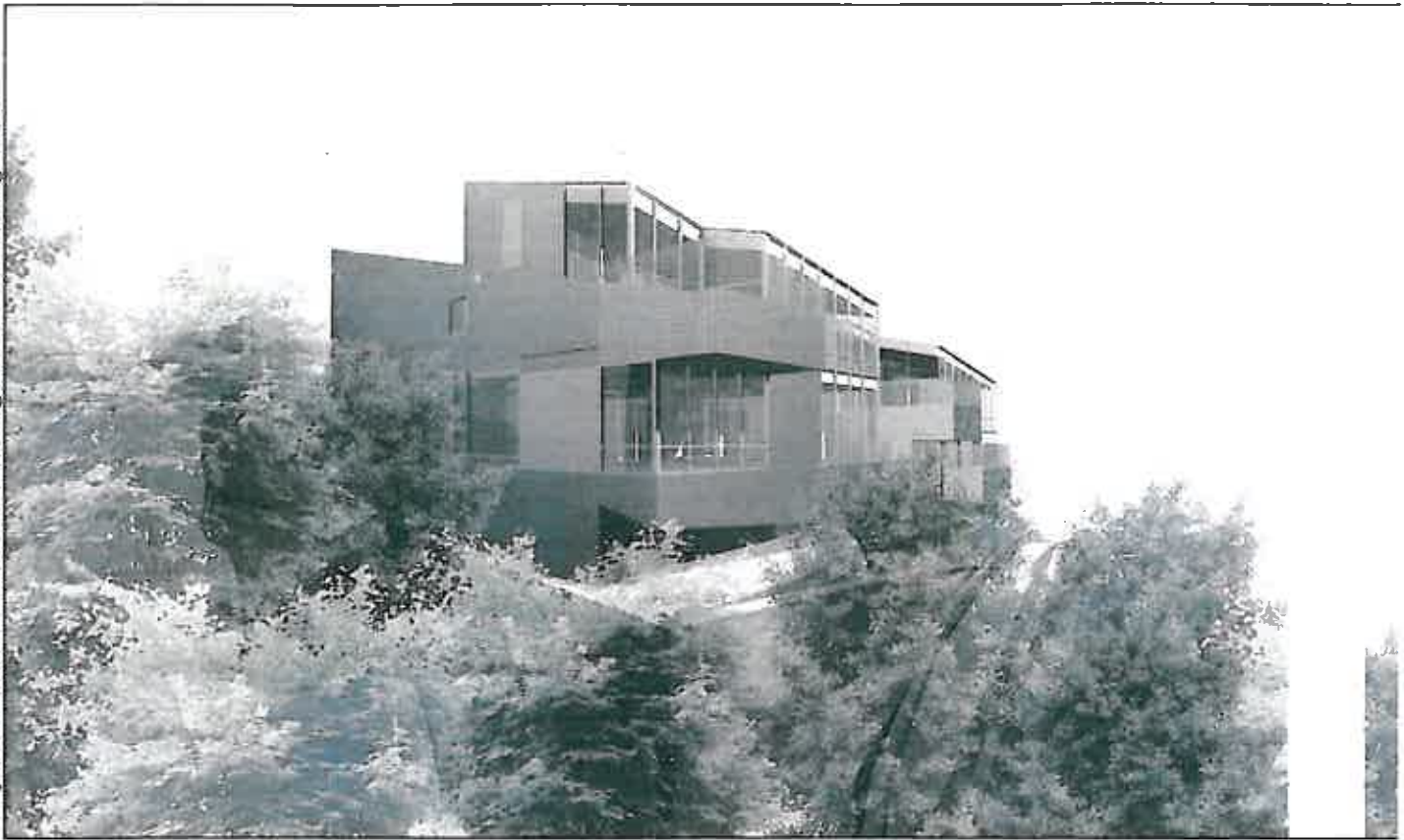
EAST SIDE(HOUSE1 UPHILL) VIEW LOOKING NORTH 2
