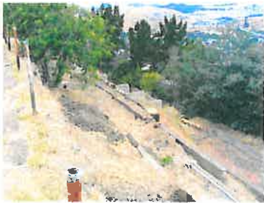
EXISTING SITE PHOTOS
