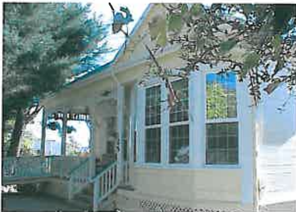
Emergency Shelter – Jackson, California Photo courtesy of Amador-Tuolumne Community Action
