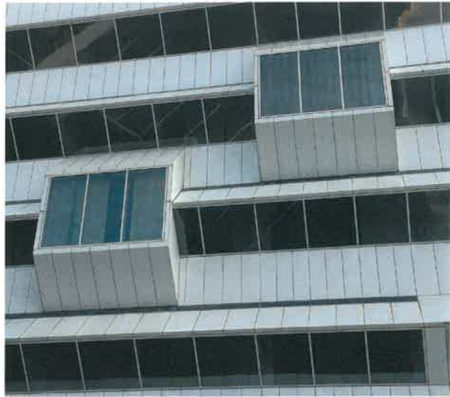
1 POP-OUT EXTERIOR VIEW - EXISTING
