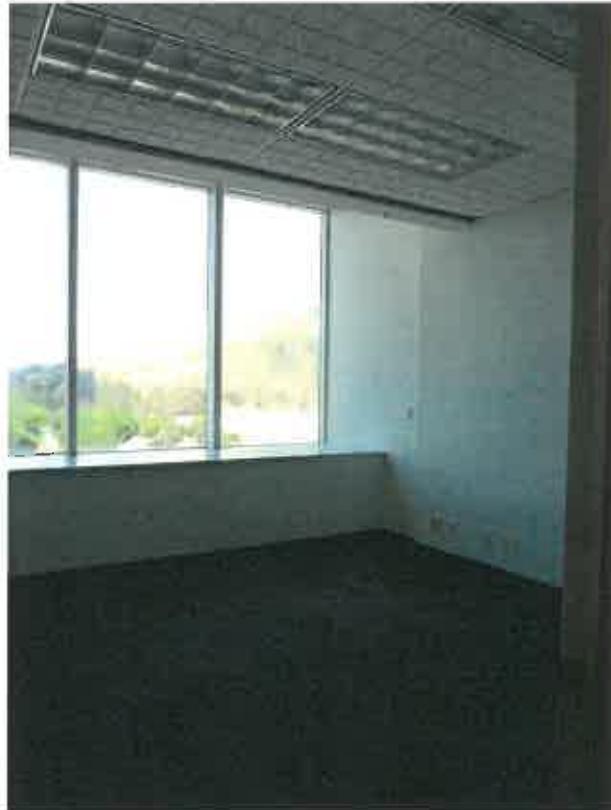
2 POP-OUT INTERIOR VIEW - EXISTING
